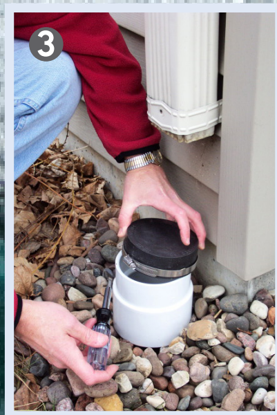
3 Cap sewer standpipe.
