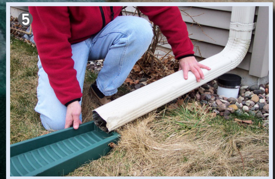
5 Attach downspout extension to elbow. Use splash board to prevent erosion.
