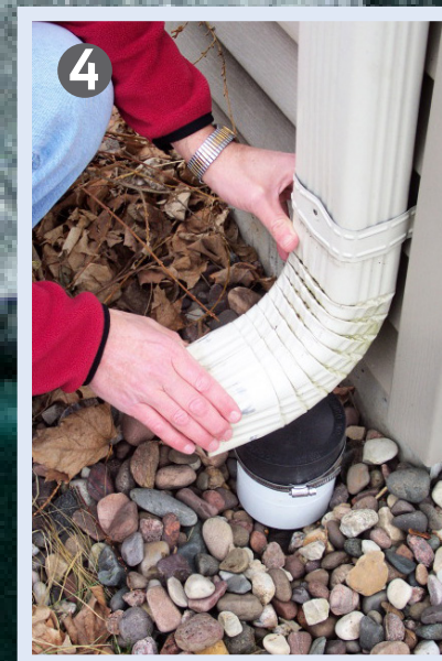
4 Insert downspout into elbow.
